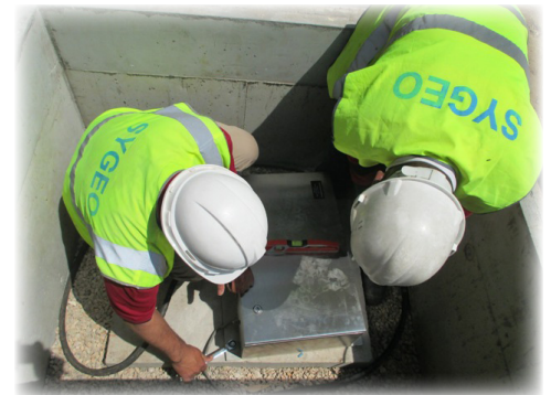
SYGEO engineers installing the seismic station.
